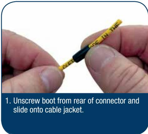
1. Unscrew boot from rear of connector and slide onto cable jacket.
