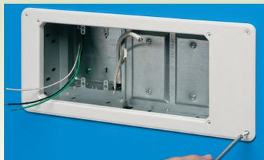
After drywall is installed, add trim plate, then install enclosure assembly to wall with outer screws.
